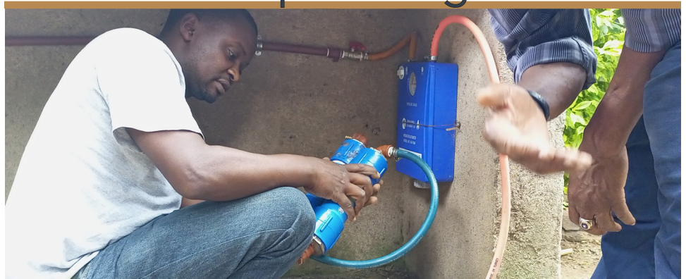
A partner organization recently invented a valve which allows biogas above the specified pressure to be released to a surplus bag. In March, the ECHO East Africa team installed 4 in the community for testing.
