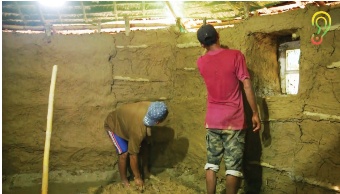
Above: Saw Shiesho and his teammates build an insulated seed storage room out of bamboo and mud. Opposite: Saw Shiesho is interviewed in front of the completed appropriate technology seed bank.
